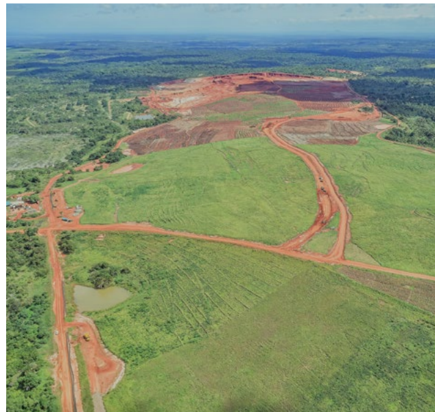
Progressive rehabilitation activities at Kwale Operations' South Dune.
