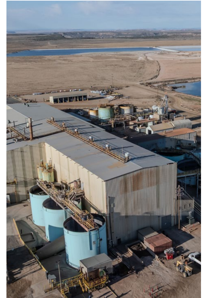
The White Mesa Mill manages uranium mill tailings and approved materials – including 11e.(2) byproduct material – in an engineered tailings storage facility designed for long-term containment and environmental protection.
