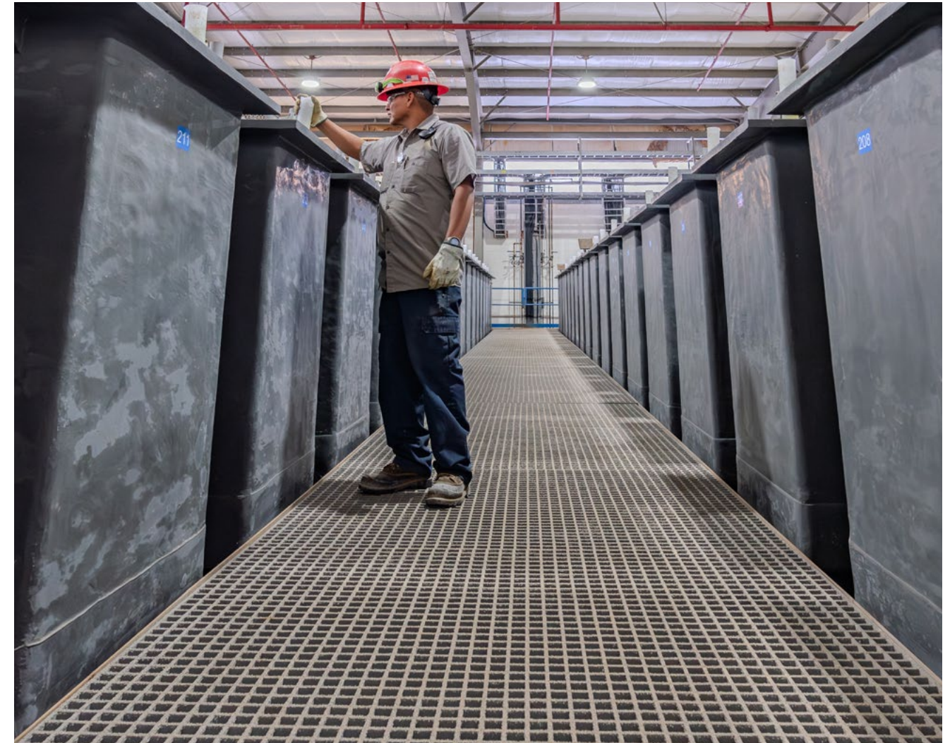
Energy Fuels employee at work inside the Mill, where critical minerals such as vanadium are processed and produced.
