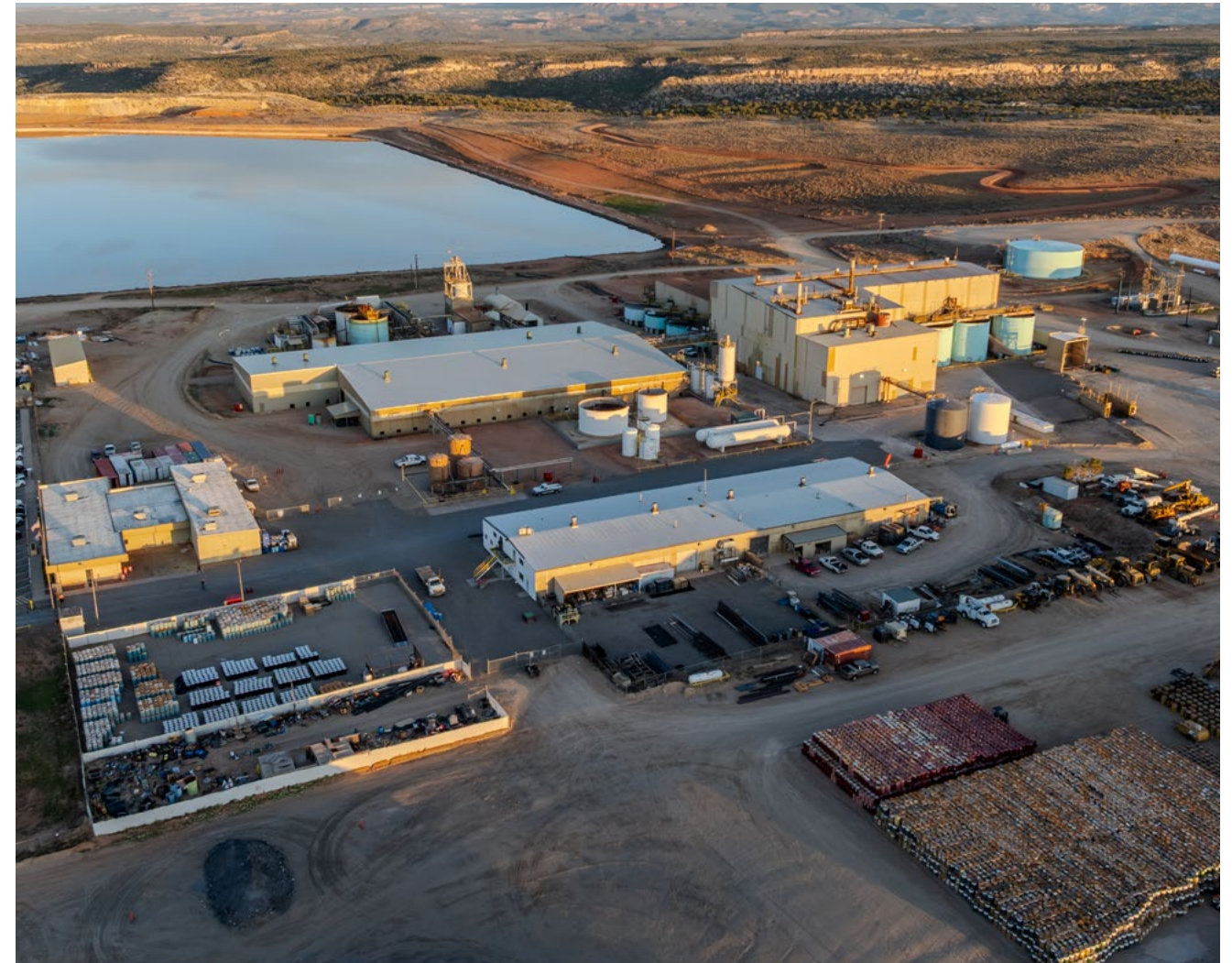
Our flagship facility, White Mesa Mill, and its evaporation pond, supporting safe, controlled recovery of critical minerals.
