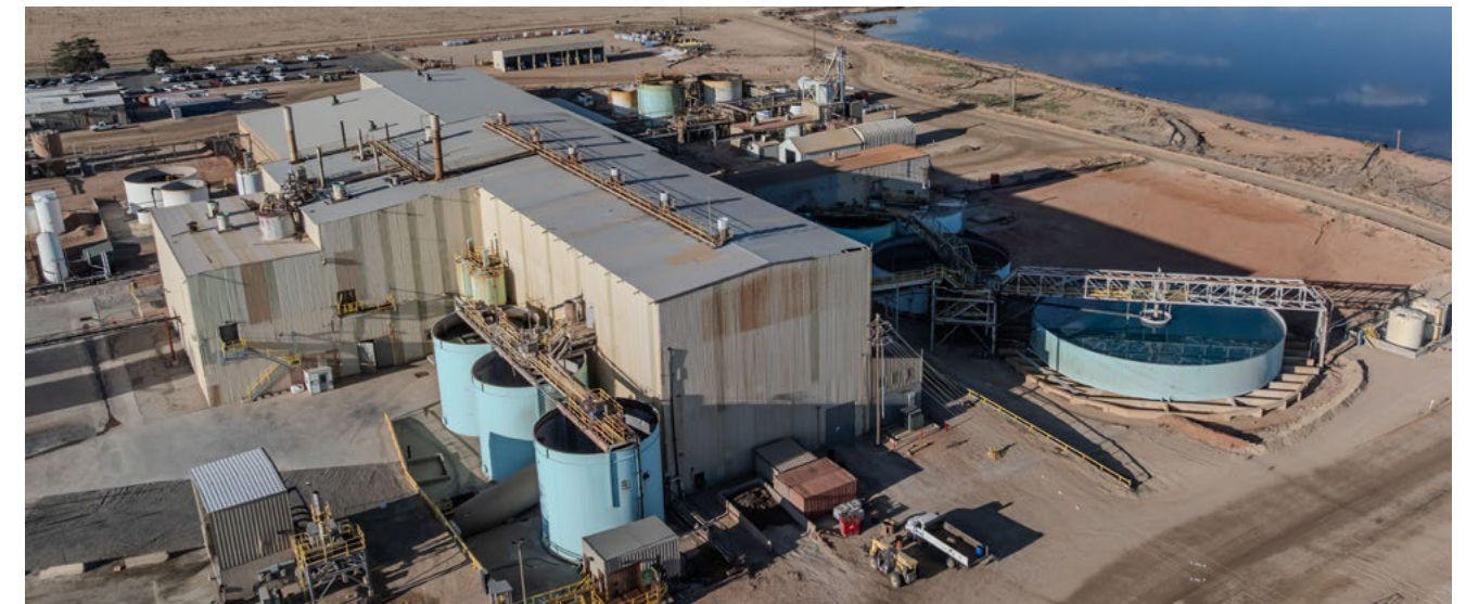
The White Mesa Mill in Utah processes uranium that supports the nuclear fuel supply chain.
