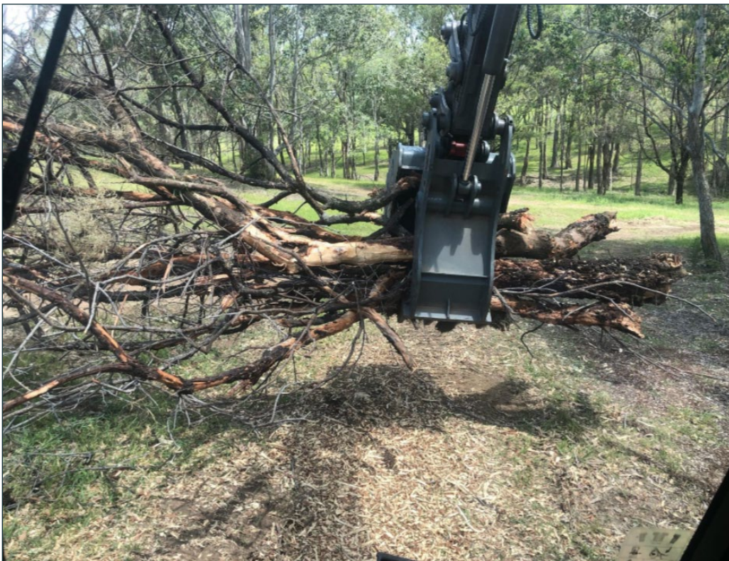
Figure 16-3: Excavator fitted with a grab attachment
